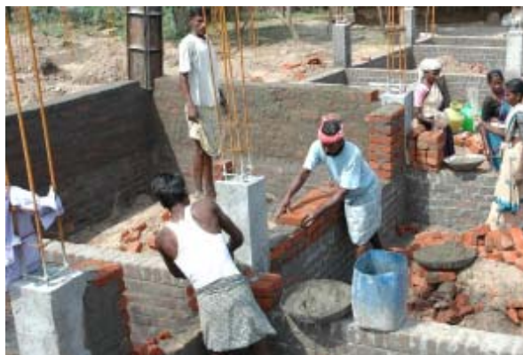
Permanent shelter construction by RDT
